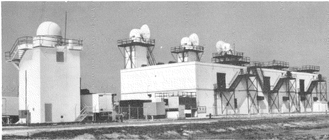
Figure 4—Range control building and phototheodolite building at site A-20. The three AN/FPS-16 radar antennas are visible on the roof.
